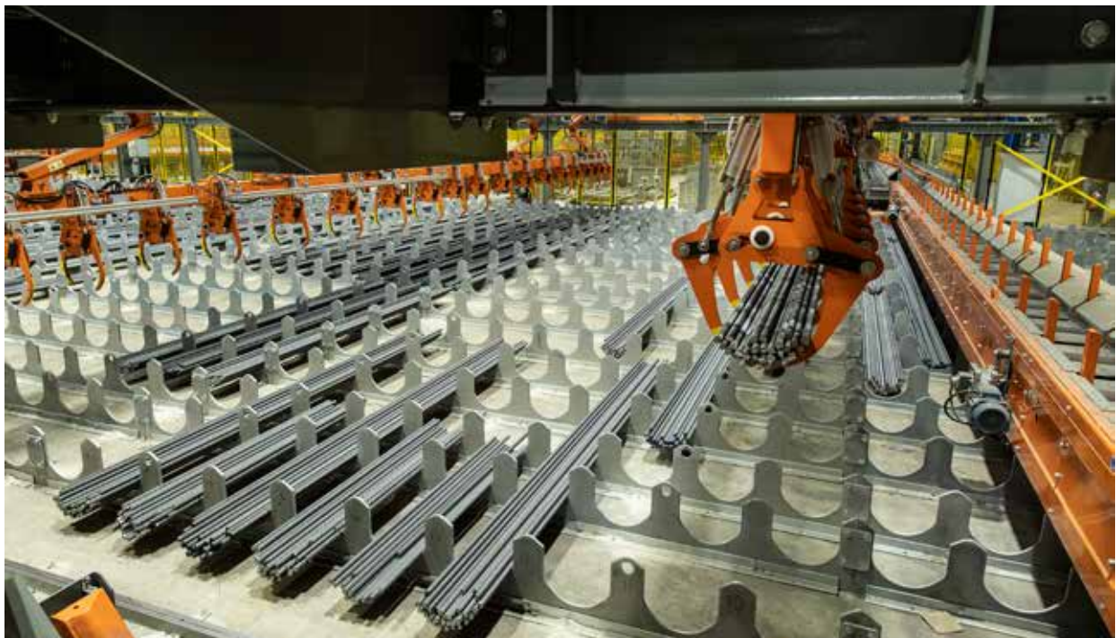
Left: work on the construction of the new headquarters of the Galeazzi Orthopaedic Institute in the former Expo 2015 site, Milan.
